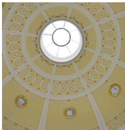
The Adam Dome, General Register House
