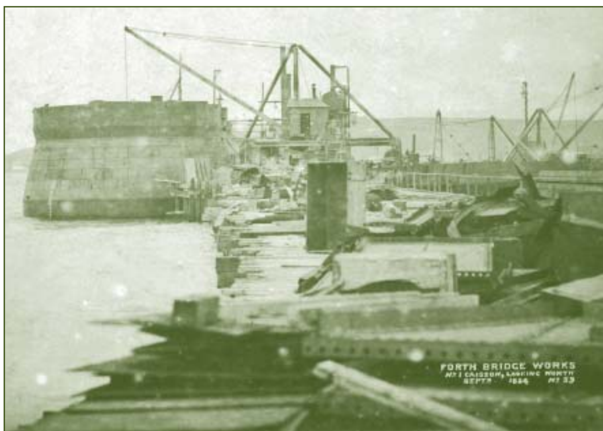
Forth Bridge Works. No. 1 Caisson, looking north, September 1884. One of the many striking images from a set of newly-acquired photographic albums showing the construction of the Forth Rail Bridge (GD1/1346/1/4).
