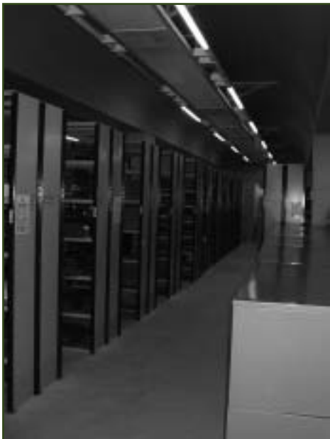
Static shelving before the upgrade programme, Thomas Thomson House.
