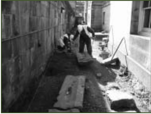
Work recommences on the east moat of General Register House, March 2007.
