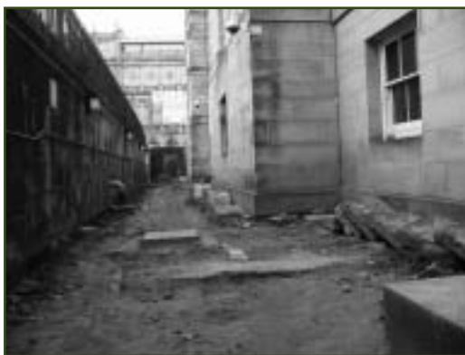
Incomplete work on the east moat of General Register House, April 2006.
